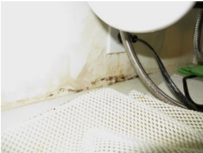
evidence of water damage noted under sink
