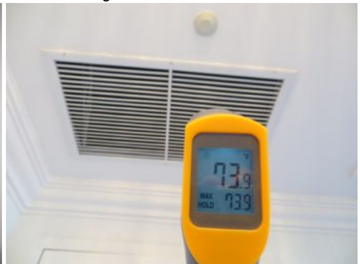
operated, Room temp ( 73°) Cold side, ( 55°)
