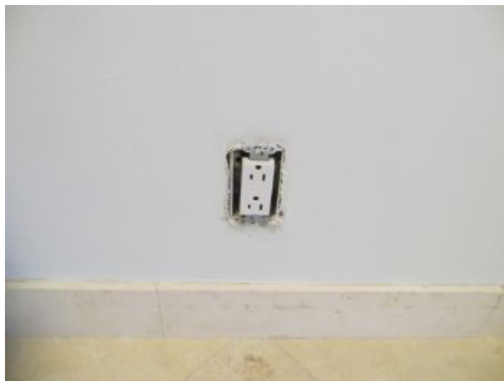
replace broken / missing outlet cover $10-20
