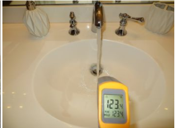
operated, ( 123°) recommend lowering temperature to between 110°-120° to prevent scalding
