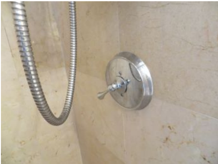
lose shower handles noted on both bathrooms, adjust $10-15
