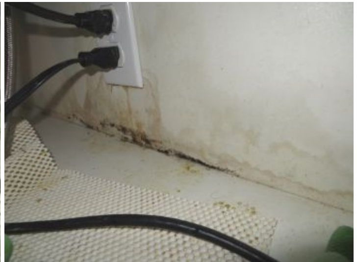
water damage under the sink, this may have an effect on cabinet structure. Recommend removing base for further evaluation
